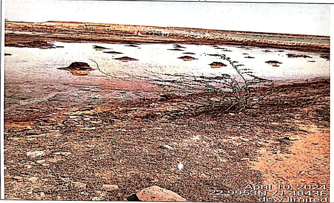
Waste water ponding (in around 20 meter * 10 meter area & 1 feet depth) located near storm water reservoir lagoon, within factory premises area
