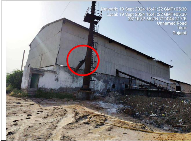
M/s. Tithi Salt (Old Name: Vidhi salt) in idle condition, Vent attached to stack is observed broken.
