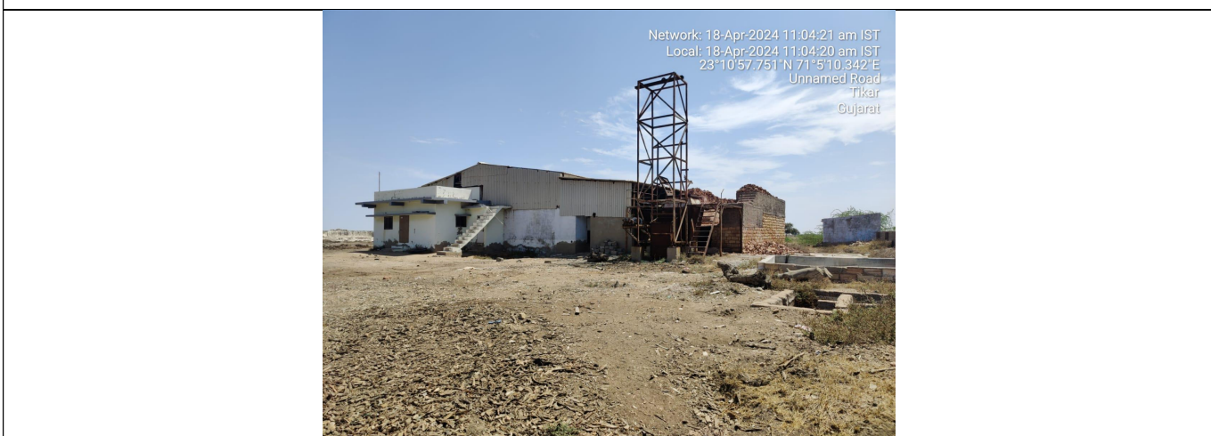
Floris Chemicals LLP - Plant and machinery removed from site.
