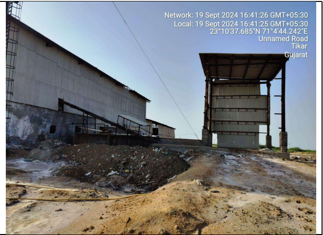
M/s. Tithi Salt (Old Name: Vidhi salt) in idle condition, Vent attached to stack is observed broken.
